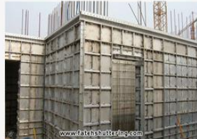
Basement Wall Plates
